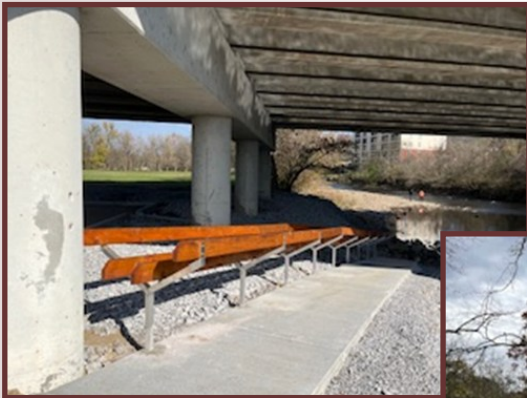
Collier Drive Blueway Landing
